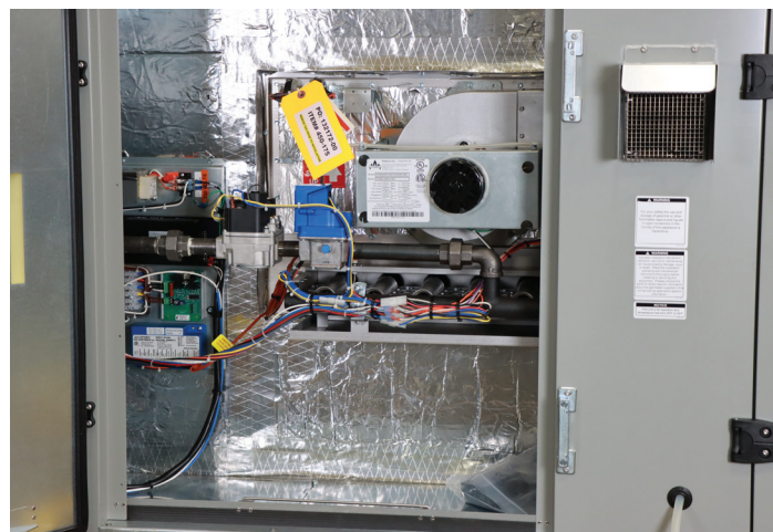
Figure 1 - Detail of Gas Heat Compartment on ExpertAire™ LCQ Series Packaged Unit
