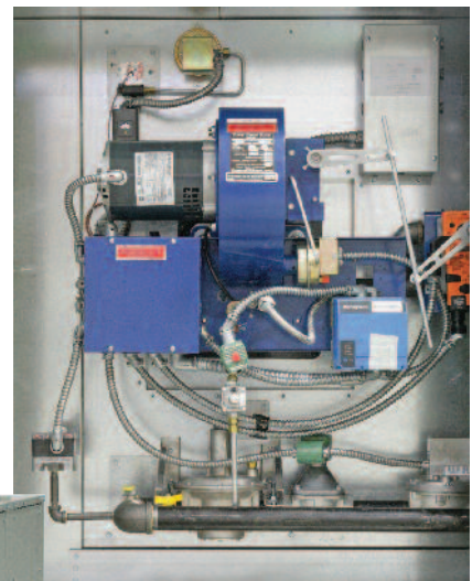
Figure 3 - Gas Burner
