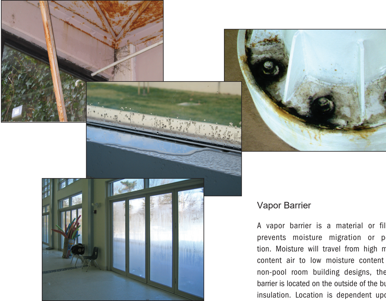
Figure 3. Examples of condensation and poor air distribution
